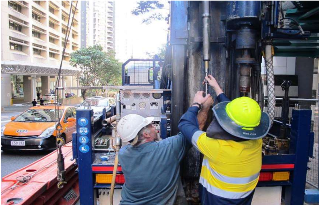
Figure 2. IST2D overcore tool about to go down the hole.
