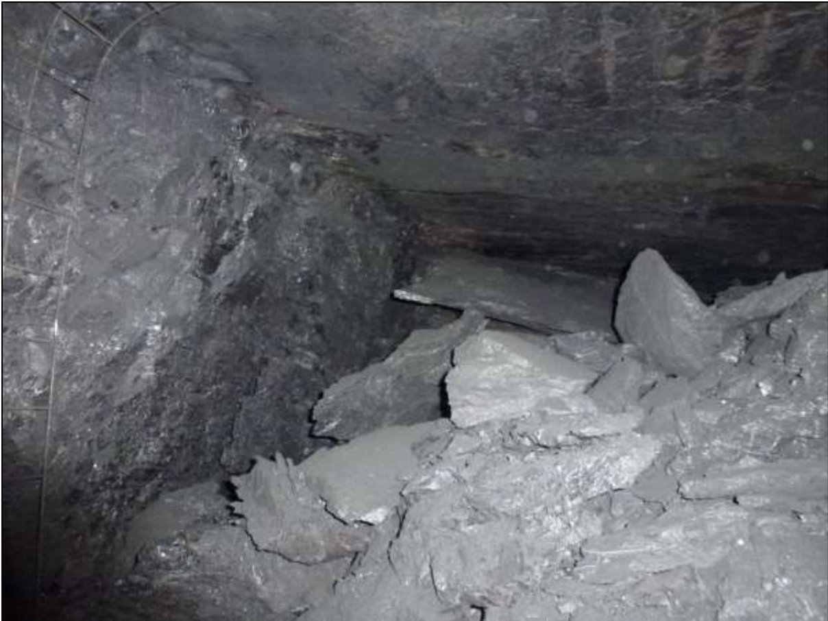
Figure 4: Photograph of a blocky burst event from the Bulli seam before clean up showing left-hand rib – face intersection
