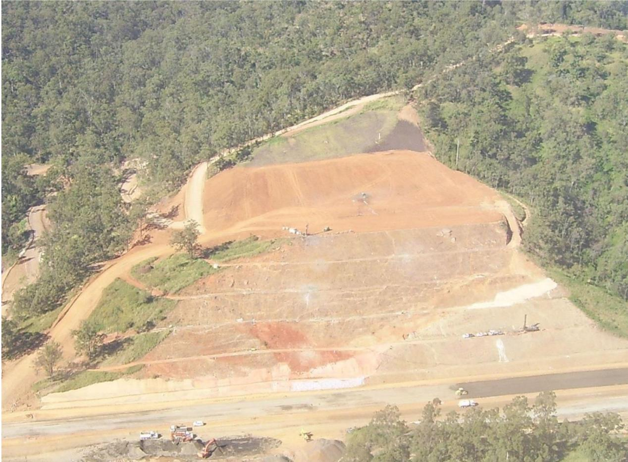
**Figure 2** Aerial photograph of cut 3 during removal of the top of the slope and filling of the toe
