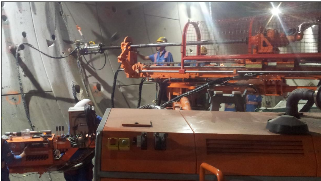
Figure 4. Drilling through a seal in a Liang Tang tunnel.
