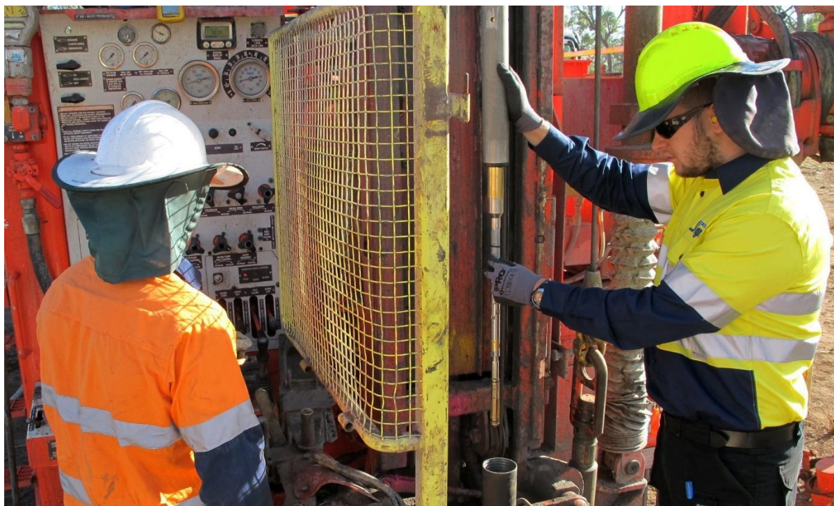
Figure 8. An IST tool being lowered into an HQ drill pipe prior to overcoring.
